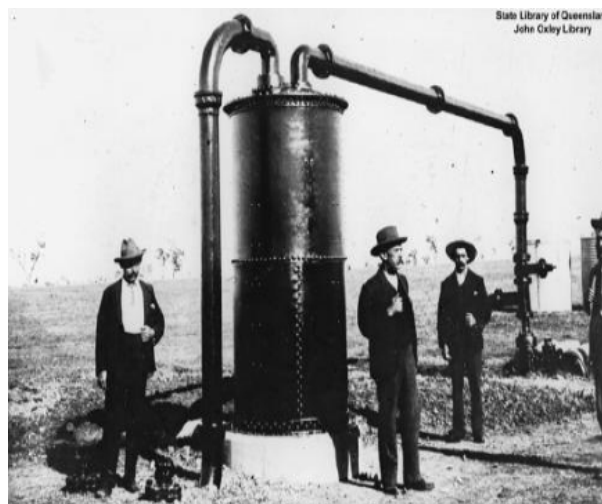
Roma gas works (ca. 1906) – plant for separating natural gas from artesian water (Source: State Library of Queensland)
